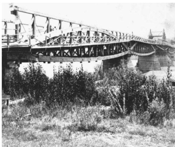
Figure 1-Timber lenticular truss bridge built in America, 1858.
