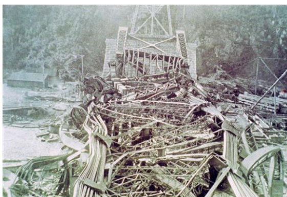
Figura 1 – Colapso da Quebec Bridge
